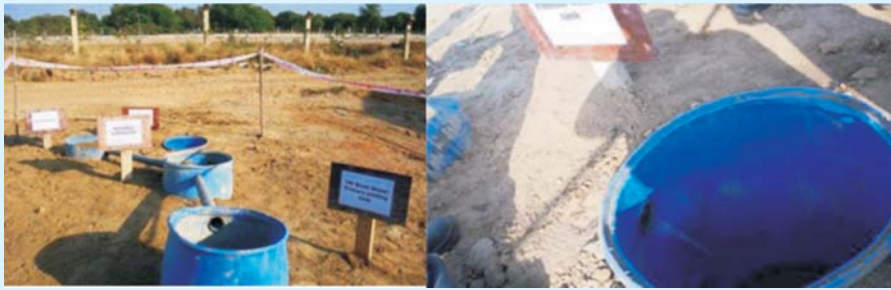
Transit mixer wash water filtration unit
