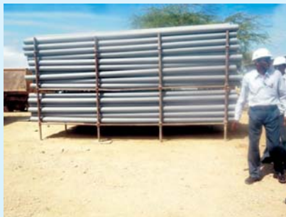
Stacking of PVC Pipes
