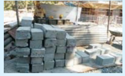
Concrete blocks made from the left over concrete from concrete mixer.
