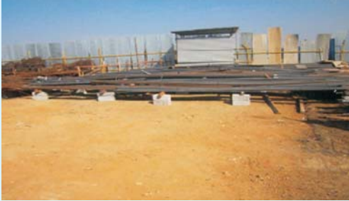
Steel reinforcement stacked neatly over sleeper
