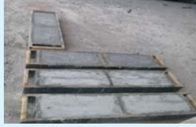
Concrete blocks made from the left over concrete from concrete mixer.
