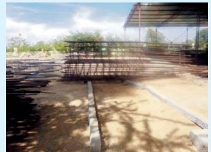
Fabricated steel stacked separately over sleeper
