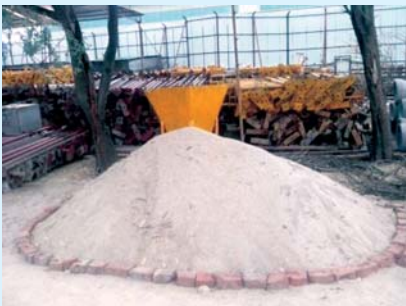
Kerb wall around storage of sand to prevent spillage
