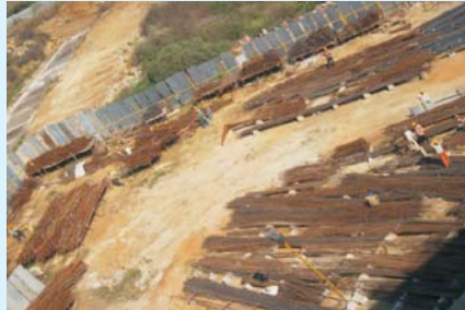
Steel reinforcement stacked neatly over sleeper
